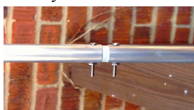
Driven Element Feed-point
